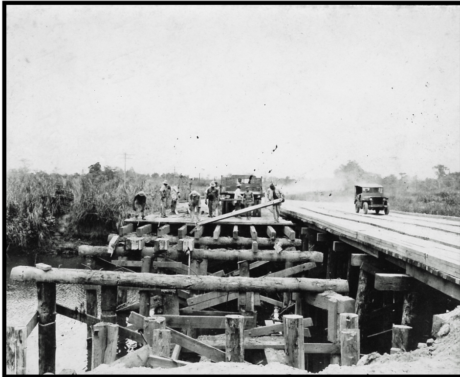
Tearing down old bridge in New Guinea
