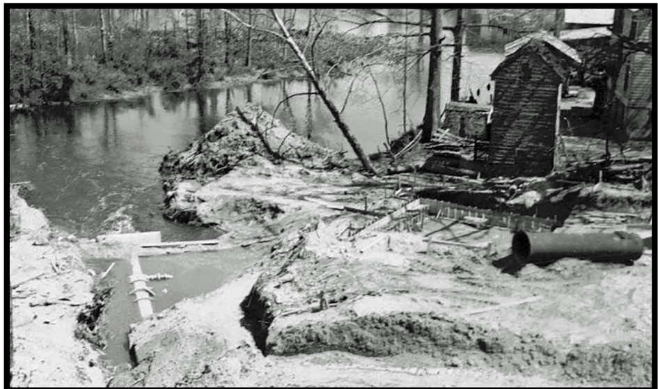
1939 Everets overlooking the creek from the west
