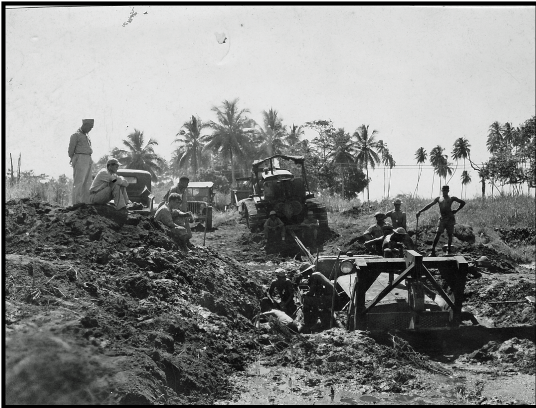
Above: Oro Bay, J. Stokes Kirk sitting on mud bank second from left with Lt. Dulac. This is a stuck D-8 Cat with four more Cat's hooked to it. It came out thirty minutes after photo taken. Below: E Company clearing road
