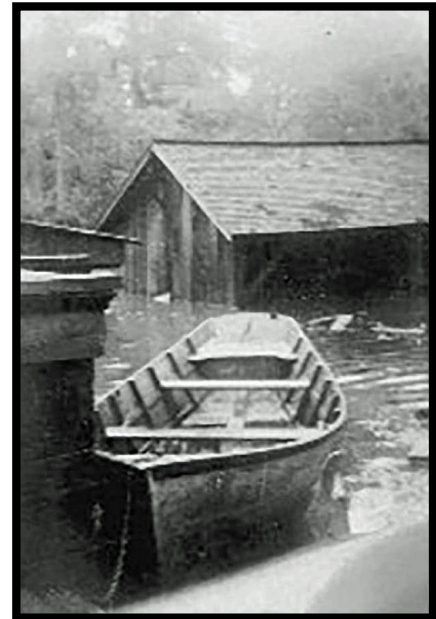
1941 Everets; Flooding in Wagner yard
