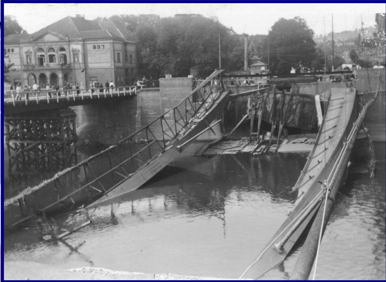
This bridge into Stuttgart is typical of German bridge demolition during retreat. Note the foot-bridge on the left which PFC Keen used many times.
